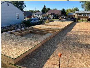
The floor joists have been installed and covered with floor decking. The east and west wall sections created at St. Paul's have been laid out in place and are covered with the sheathing boards. When they are finished, they will be stood up and the north, south and interior walls will be installed.
