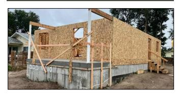
The Habitat house is progressing. The exterior walls that were made at St Paul's are in place and most have the chipboard exterior sheath attach. The interior walls are stacked inside waiting to be stood up and secured to the exterior walls. Soon we will see the roof trusses in place.
