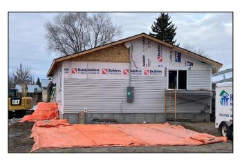
In the front the new sidewalk and front steps are poured and curing under the orange blankets. The blankets should be able to come off by Friday.
