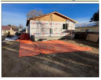
In the backyard of the Habitat house, the sewer and freshwater connections have been made and buried. Preparations are made for a 20' x 20' concrete pad and sidewalk going to the house. Orange tarp keeps the dirt dry and warm before the concrete. The concrete pour will include the slab, two outside stairs and replacing the front sidewalk along 18th St.
