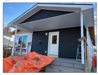
The front porch area with its gray accent color is finished and now they're working on the siding on the front of the house. Note the orange tarp covering the forms for the front steps.
