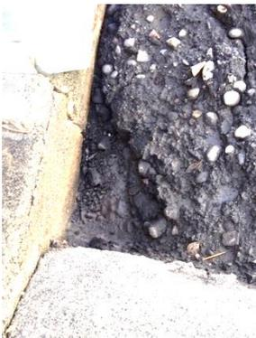
identified a hole in the asphalt that was letting the rainwater enter. It flowed under the outside stairs and into the boiler room hallway. Rob has filled up the hole with asphalt patch, and built-up the area to cause the water to drain away from the building. He also sealed the cracks in the asphalt, just to be sure. Once again, Rob to the rescue.
